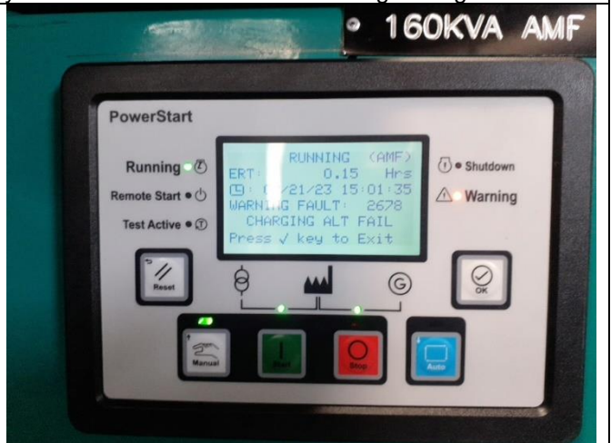
Generator Set 160 kva during testing panel display
