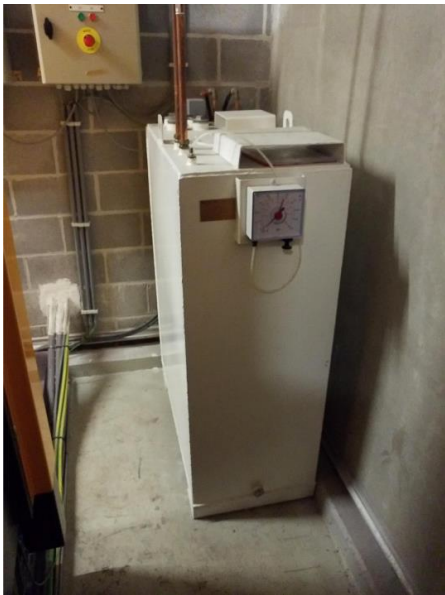
Tank to disconnect, recuperation of fuel, dimount
